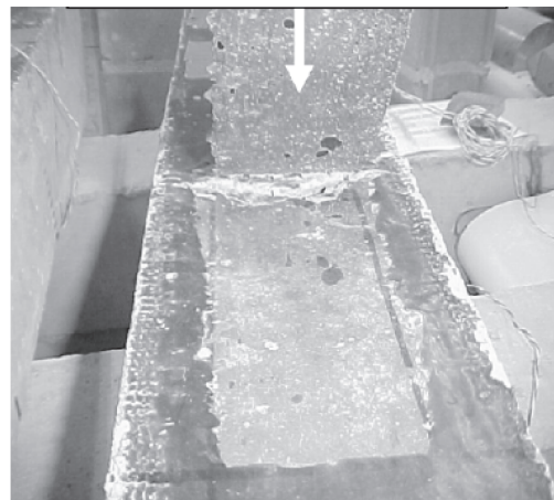
Figure 4. It polymeric resin used as protection against the corrosion [50].
